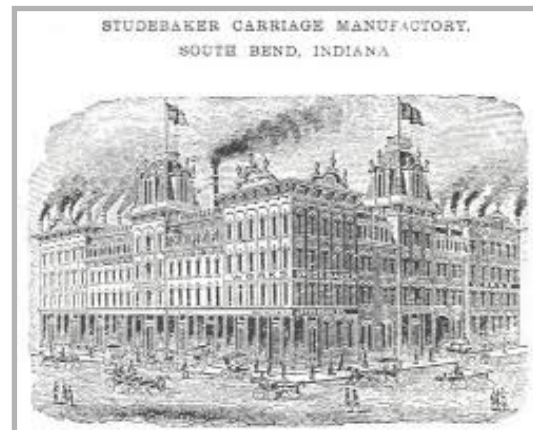
Studebaker Factory 1874, Rebuilt
